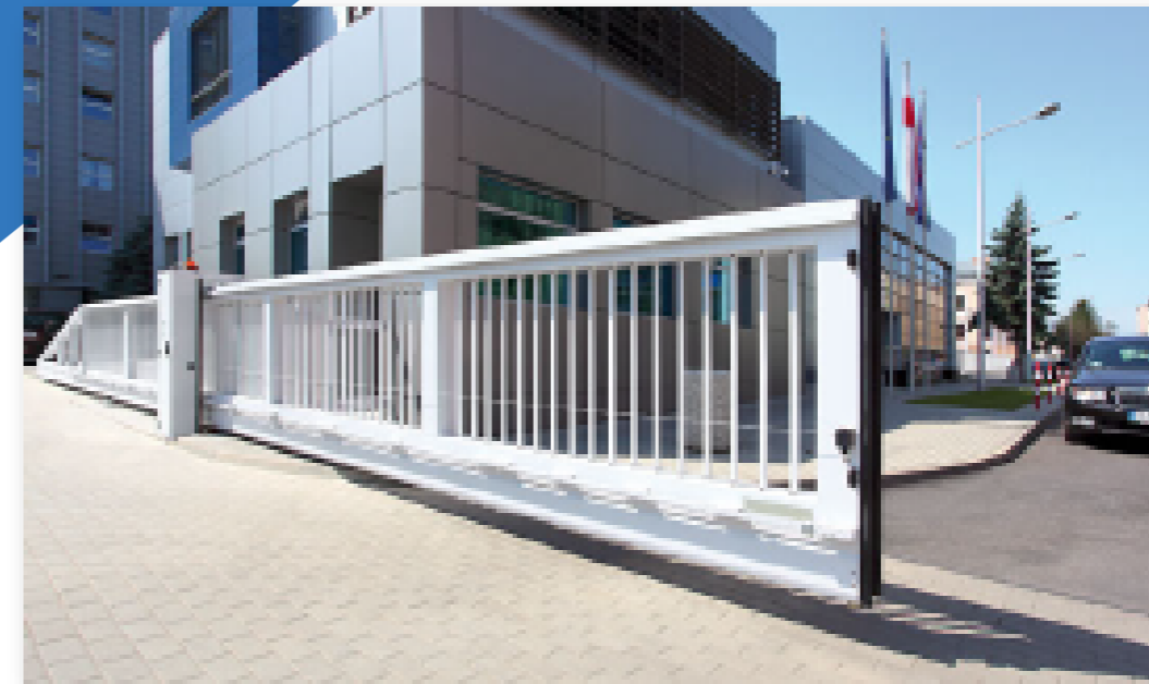
▲ Cantilever Sliding Gates
